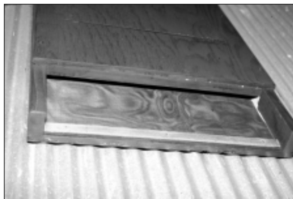
In this chamber, 7/8" in height, a fiberglass window screen is stapled to one internal side that extends down about 5" and serves as a landing strip. The unpainted wood cleat at the bottom of the screen holds the screen tight. It also serves to evaporate urine, thus preventing urine running down the side of the building.
