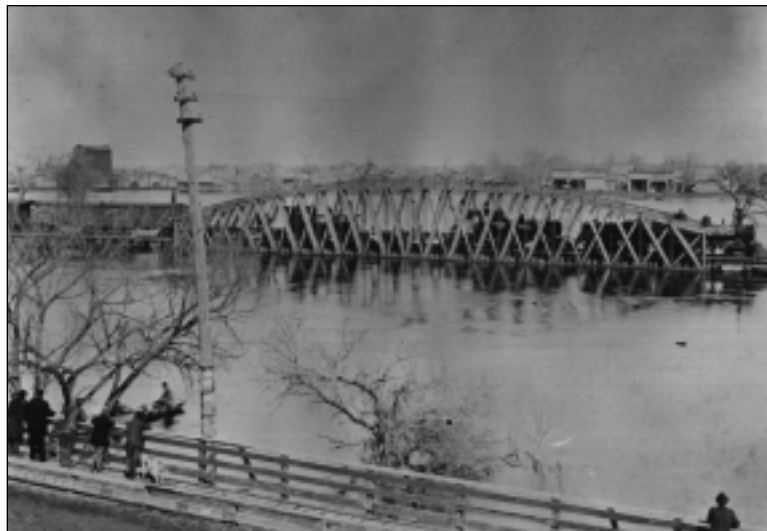
This is the Red River at high water flood stage in Moorhead in 1882. A Northern Pacific Railroad train has been driven onto the bridge to prevent it from being washed away. (Originally published in Roots, Spring 1978.)
