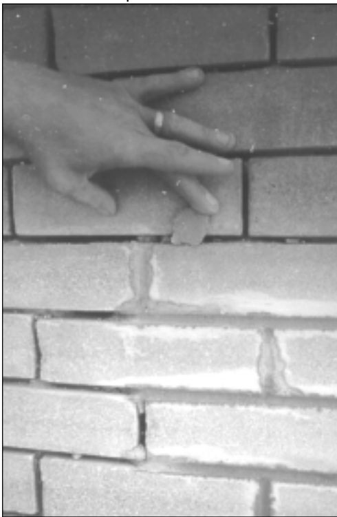
Above: A sample of mortar is being matched with the historic mortar; just below it are profiles of "finger joints" made by striking the mortar with the finger.
