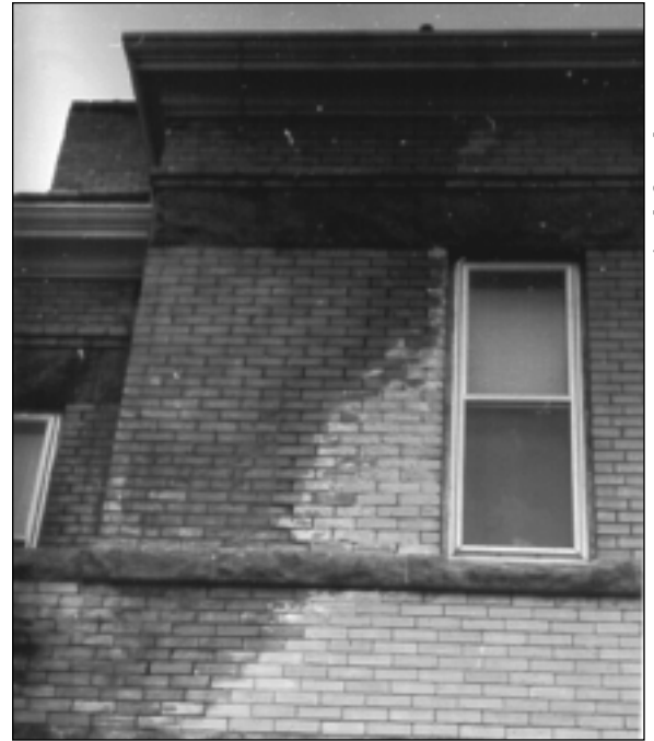
This photograph shows damage to mortar and masonry caused by a leaking gutter.
