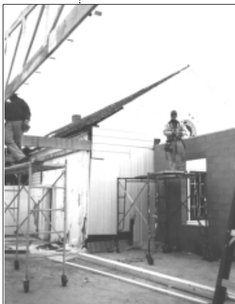
This photo, taken Nov. 20 from inside the former meeting room, shows the new north wall (right) and the first new rafter. The men are from Nelson Construction Co.
