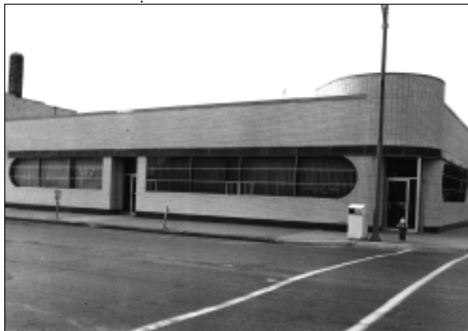
Above: the Greyhound Bus Depot in Brainerd, Crow Wing County, built ca. 1950. It is a good example of the streamlining found in Art Moderne buildings.
