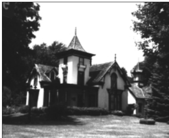
The Nicollet County Historical Society received a grant for restoration work at the Eugene St. Julien Cox House in St. Peter
