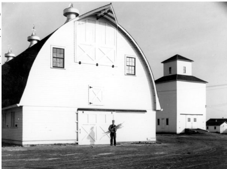
Red River Valley dairy barn, Cass County, North Dakota, 1940. From the traveling exhibit "Barn Again!"
