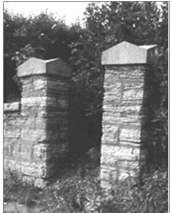
Two limestone gate posts in St. Paul, built around 1885.
