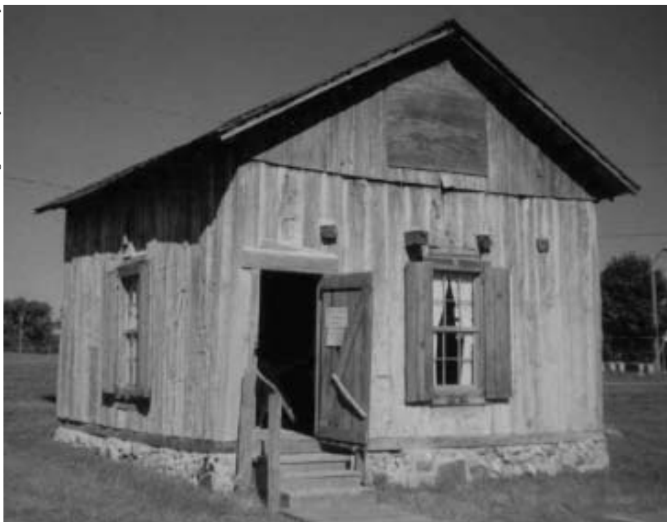
The Bonk-Ailsleiger Cabin, of vertical log construction, stands on the Wright County Fairgrounds in Howard Lake. It will be interpreted to the period 1880–1900.
