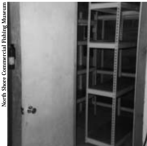
An enclosed room will provide locked, environmentally controlled storage for the North Shore Commercial Fishing Museum's collection of photographs and artifacts.
