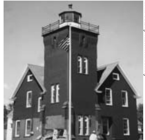
The reroofed Two Harbors Light Station awaits completion of a new paint job.
