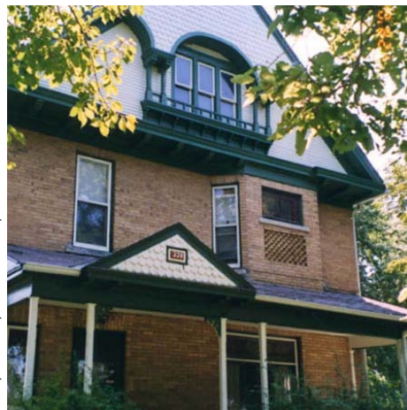
An infusion of funds from the City of Willmar has helped the Kandiyohi County Historical Society renovate the 1893 Sperry House. Reconstruction of the front porch will add the finishing touch.
