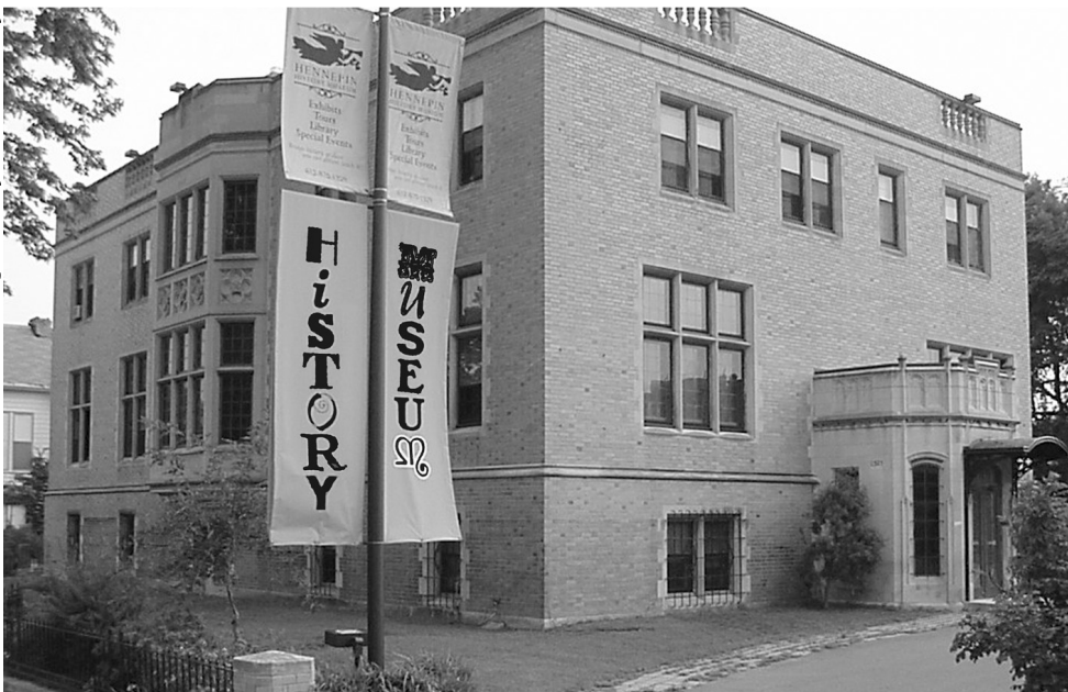
CAP assessors recommended masonry repairs and humidity monitors for the Hennepin History Museum but cautioned against installing a modern HVAC system in a historic building not designed for it.
