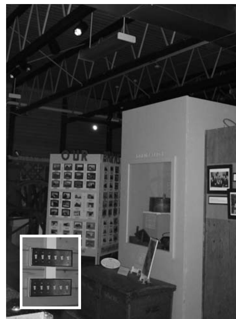
A lineup of switches and dimmers (inset) controls 12 circuits of new track lighting at the Kandiyohi County Historical Society. Old fluorescent fixtures will be removed.
