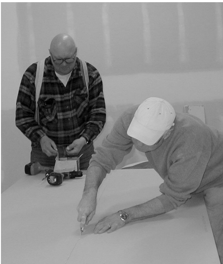
Board members Dick Hanson (left) and Peter Reis pitch in on construction of the White Bear Lake Area Historical Society's new storage space at City Hall.
