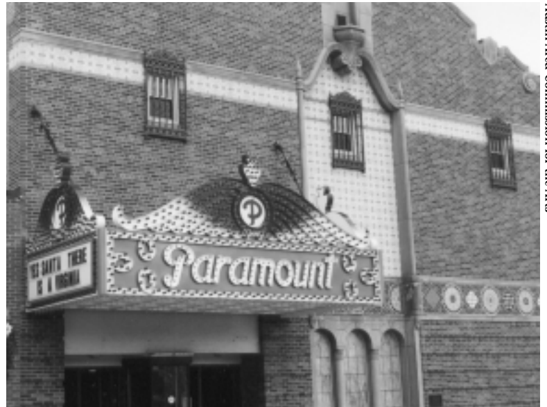
The Paramount Theatre’s new marquee, recreated from historical photographs, was funded by a local donor.
