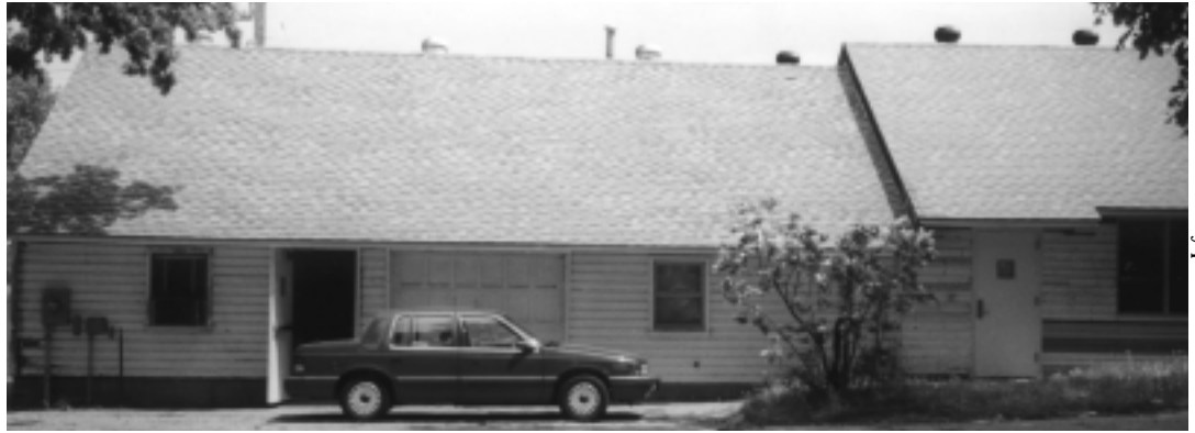
Structural problems slowed work on the Richfield Historical Society's facility. A new roof and HVAC system are in place. Still to come: new siding.
