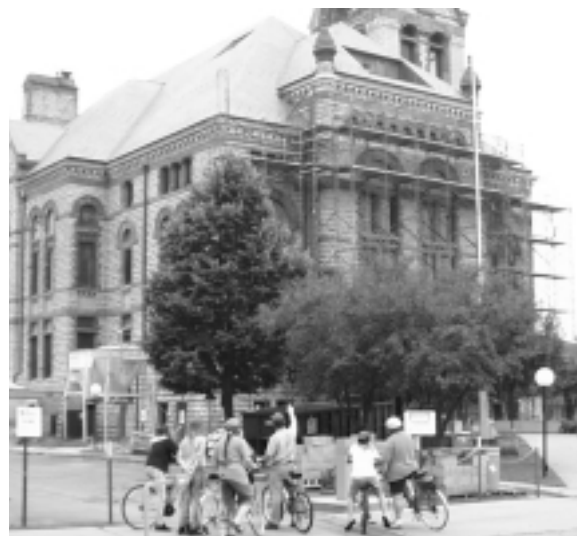
Mark Peterson, executive director of the Winona County Historical Society, points out restoration work on the county courthouse during a "Bike, Skate and Scooter" tour of Winona.
