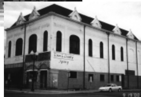
In 1892 (above left) the St. James Opera House building housed a bank on the ground level and the opera house above. A 1950s alteration bricked over the storefronts and covered the upper story with paint. Last year restorers began uncovering the original arched entrance (above right).
