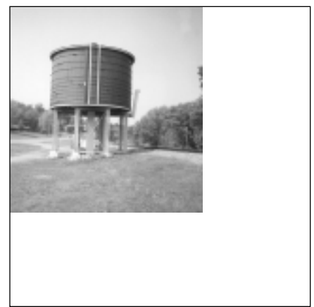
The Carver Water Tower, as it looked after restoration. The railroad tracks are to the right.
