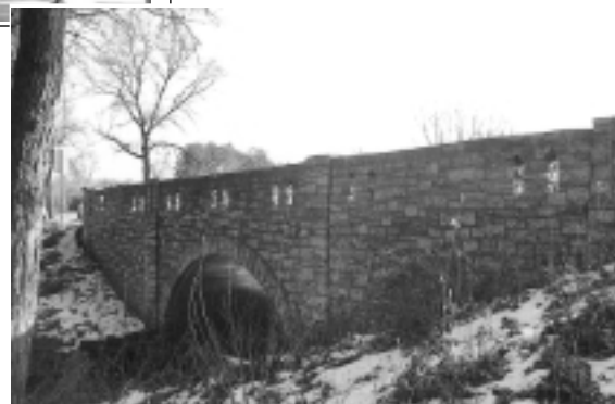
Bridge No. 8096 (below) in Northfield was originally built in 1918 as a reinforced-concrete arch with a 22-foot roadway. In 1947, the bridge was doubled in width and covered with roughly coursed, rock-faced limestone detailed in the Late Gothic Revival style. The bridge is eligible for the National Register for its architectural design and workmanship.
