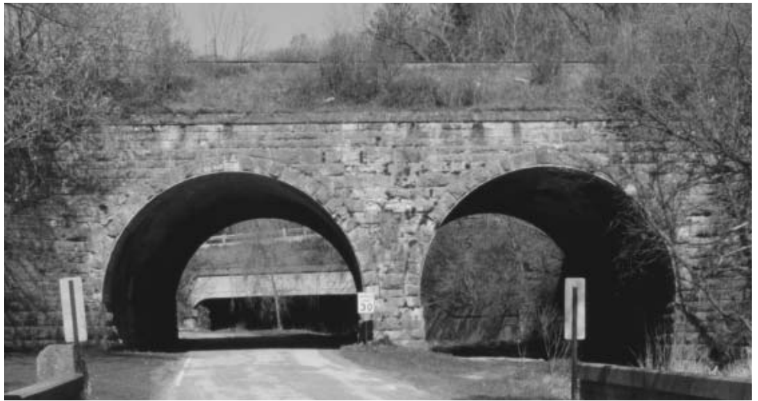
This 1882 stone arch bridge in Winona County is one of many in the DM&E Railroad corridor.
