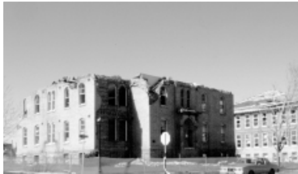
St. Peter Central School, above, in 1980; below, a few days after the March 29 tornado.
