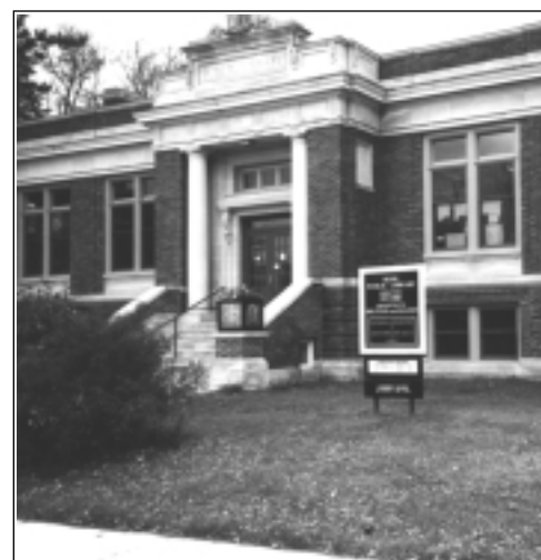
Above: New energy-efficient windows that matched the originals were installed on the Buhl Public Library (1917) in St. Louis County; funds from the MHS State Grants-in-Aid program were used.
