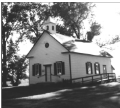
Above: Several projects were completed on District No. 48 School (1870) in Collinwood Township, Meeker County, including: installing new double-hung sash and storm windows, constructing a new roof, replacing deteriorated siding, repair and re-installing original shutters, and painting both the interior and exterior of the building. Funds were provided from the state bond-funded County and Local Preservation Project Grants-in-Aid program.
