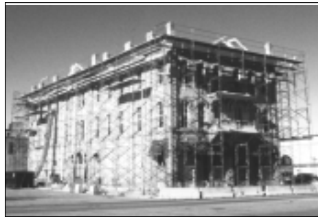
The Nicollet Hotel, listed on the National Register of Historic Places, sustained major damage. The new owners who acquired the building following the storm expect it to reopen in the spring.
