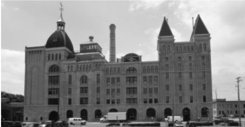
The Minneapolis Brewing Company complex in northeast Minneapolis, built during the 1890s, has found new use as architectural offices. It will also soon be home to the Pierre Bottineau Branch Library.
