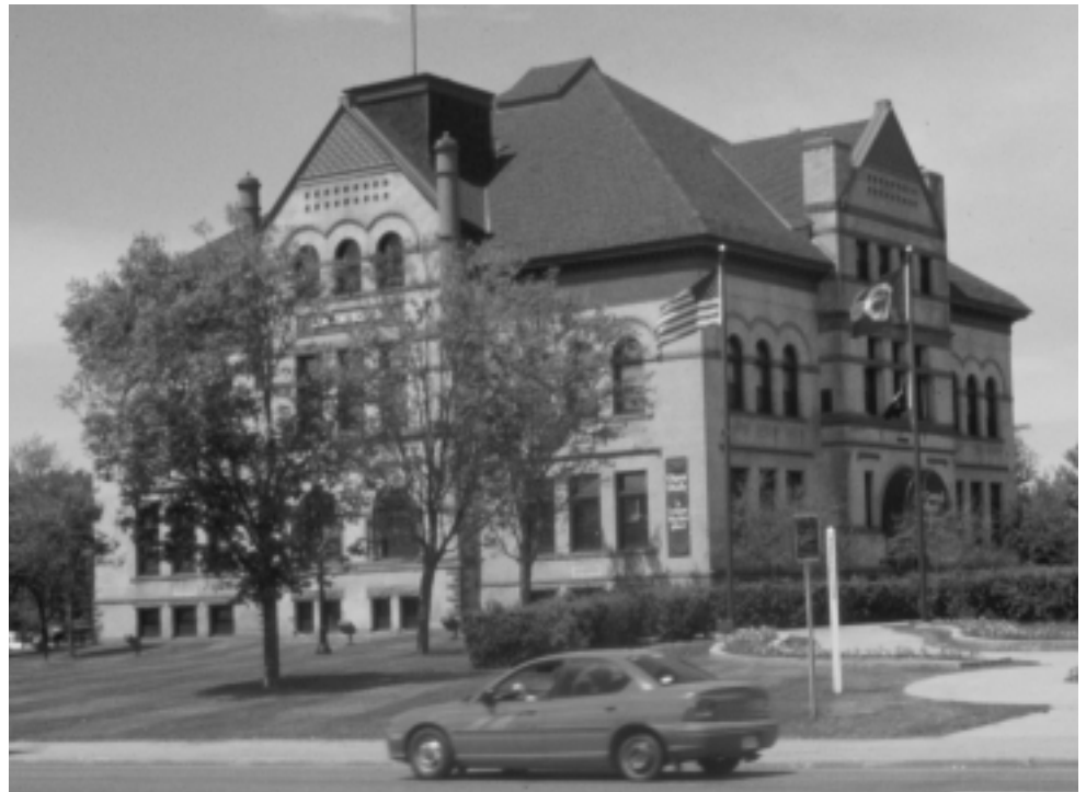
Central School in Grand Rapids, built in 1895, will be repointed with funds from a capital grant.
