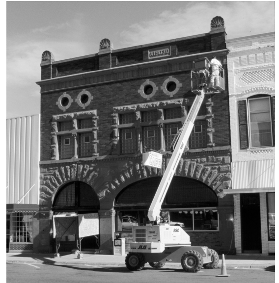
Restoration work on this commercial façade in Todd County's Long Prairie in 2001 included masonry repairs.
