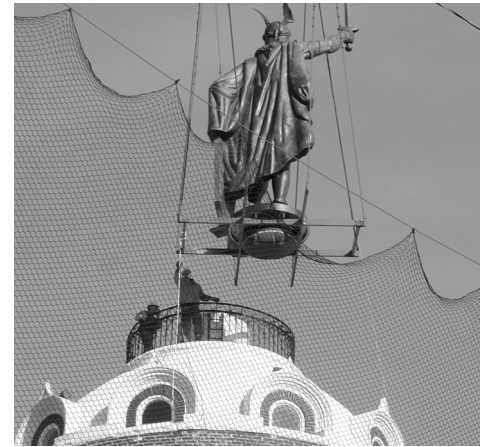
Left: The Hermann Monument before rehabilitation. Right: The restored statue is hoisted back into place.
