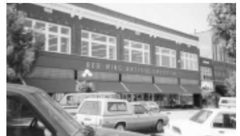
Before (top): The brick façade of the Goodhue County Cooperative Company Store had been completely obscured by 1960s-era metal panels. After (bottom): Extensive rehabilitation work restored the building to its original appearance.
