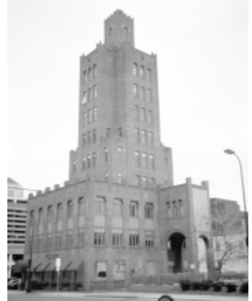
Despite its historic designation, the vacant Ivy Tower (Second Church of Christ, Scientist Administration Building, 1930) in downtown Minneapolis has deteriorated after years of neglect. Under the city's new historic preservation ordinance, city officials have the legal authority to require owners of historic properties to maintain them.
