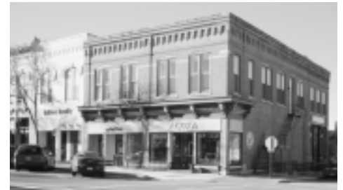
Holland Block Building, Northfield after rehabilitation.
