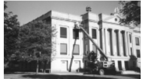
Workers repoint the Lincoln County Courthouse during its rehabilitation.
