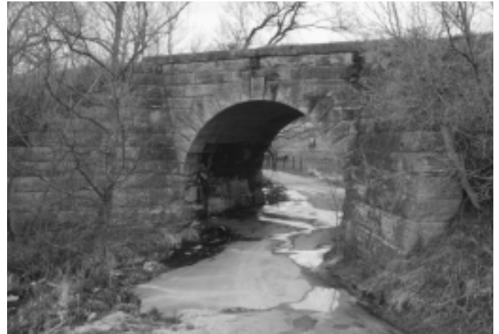
This 1910 stone arch railroad bridge in Eyota, Olmsted County, is one of hundreds in the path of the proposed DM&E corridor.
