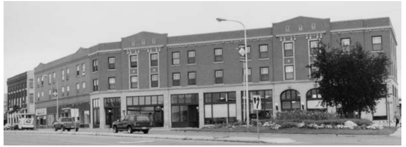
The Graystone Hotel (1916 -17) in Detroit Lakes was rehabilitated with federal preservation tax incentives for commercial and residential use.
