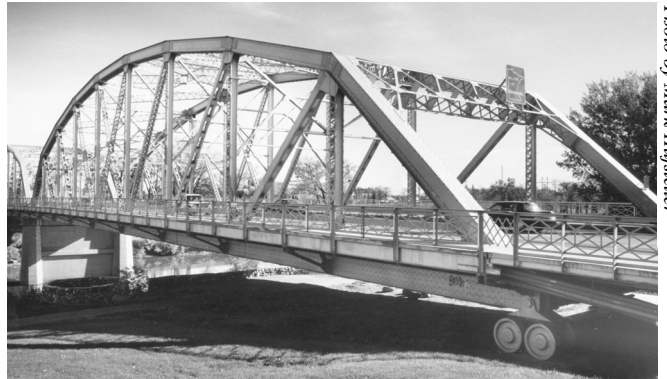
An expansion-bearing system featuring frames of wheels on pairs of track castings enabled the Sorlie Memorial Bridge (1929) to compensate for motion caused by unstable ground.
