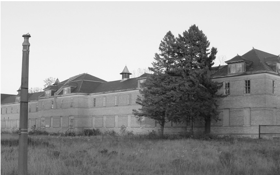
Long vacant, the buildings of Fort Snelling's Upper Post are in various states of decay.
