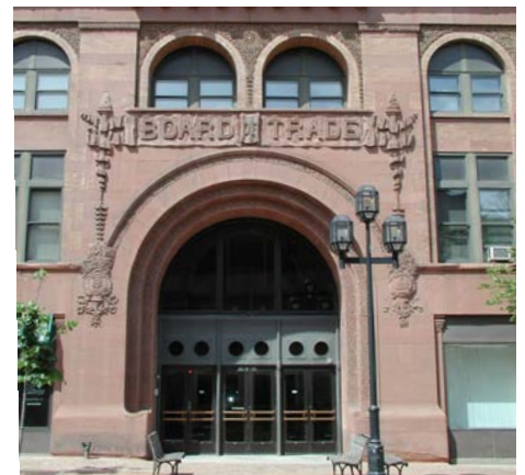
From the 1880s to the 1920s, Duluth was one of the nation's premier timber-processing centers and a major port for grain and ore shipping. Reflecting this industrial past is the city's Commercial Historic District, containing 107 buildings, among them the Board of Trade, that represent commercial adaptations of popular architectural styles of the day.
