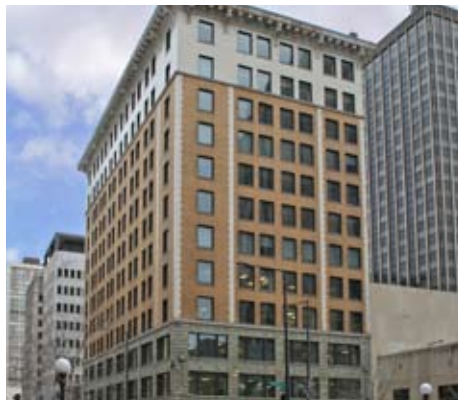
The 12-story Commerce Building served as headquarters for the Commercial Club of St. Paul and offices for the St. Paul Association of Commerce - among the first such organizations in the country to join forces in a modern skyscraper in a key downtown location. Both organizations were leaders in the city's efforts to support economic growth.
