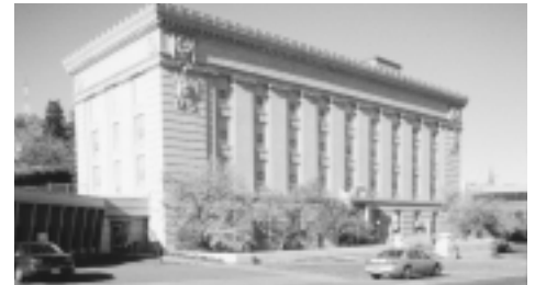
The St. Louis County Jail (1924), part of Duluth's Civic Center complex, was the subject of a 1999 reuse study.
