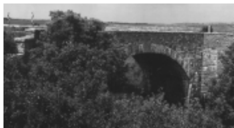
Split Rock Bridge, Eden Township, Pipestone County.
