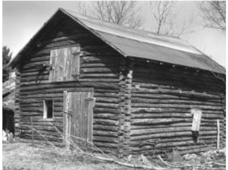
This horse stable is one of several buildings on the Pyhala Farmstead in St. Louis County to be restored with a capital grant.
