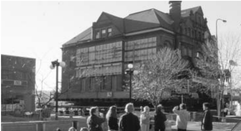
Spectators watched as the Armstrong House inched along St. Paul's West Seventh Street. Now on a new foundation in the locally designated Irvine Park Historic District, the house will undergo rehabilitation by the city and conversion to condominiums.
