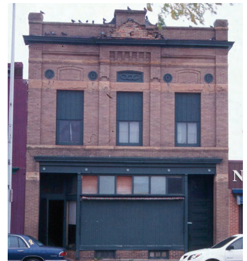
New Richland’s Strangers Refuge Lodge No. 74 (IOOF), built in 1902, will be rehabilitated using funds from a capital grant.
