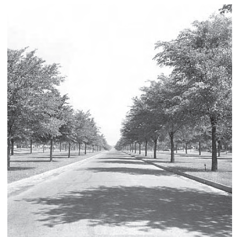
Part of Minneapolis's Grand Rounds, Victory Memorial Drive (shown here in 1945) accommodates cars, pedestrians and bicycles.
