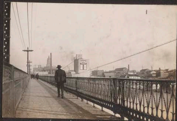
Wabash River Bridge
