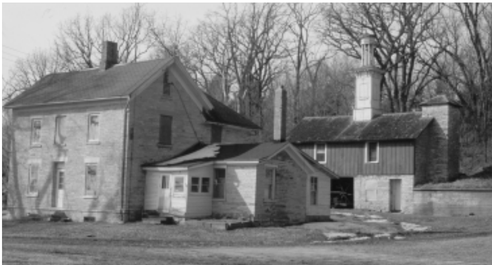
The Olmsted County Historical Society will use its grant-funded historic structures report to guide restoration of the 1860s George Stoppel Farmstead near Rochester.
